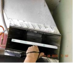
10.1.2 Filter Cover Does Not Fully Secure
